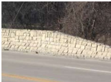
Bridge facing along River Road
