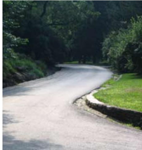
Private Drive with Stone Curbing
