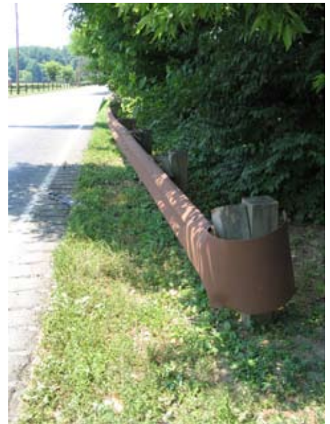
Cor-ten Guard Rail on River Road
